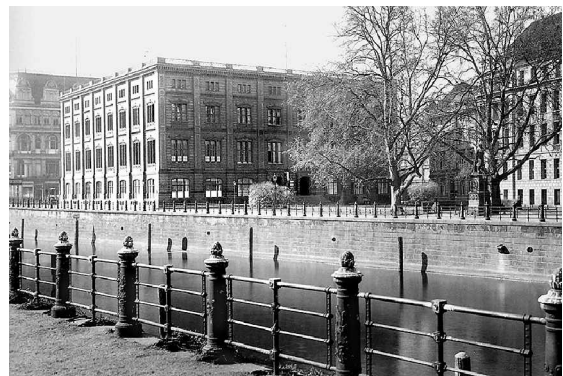
Bauakademie, Photograph 1930 (source: Institute for the Photographic Surveyance of Buildings)
